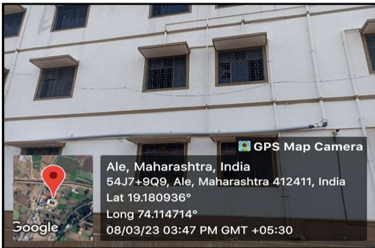
Water distribution system in the Campus
